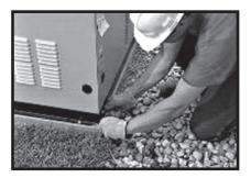
Connect an approved ground strap to the grounding lug on the base frame and to an approved earth ground or grounding rod as specified by local regulations.
